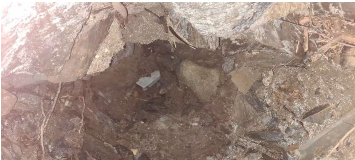
Figure 2: Void (Fig. 1) interior.
