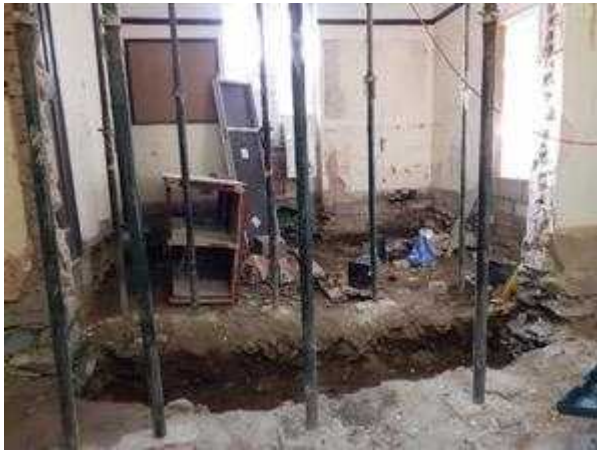
Excavations underway and doorways being blocked up
