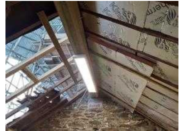
A second layer of roof insulation was installed.
