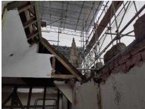
A temporary roof was constructed. The ridge slates and tiles to the roof to the police station were set aside for reuse. Ceiling timbers were replaced, secret gutters were formed.
