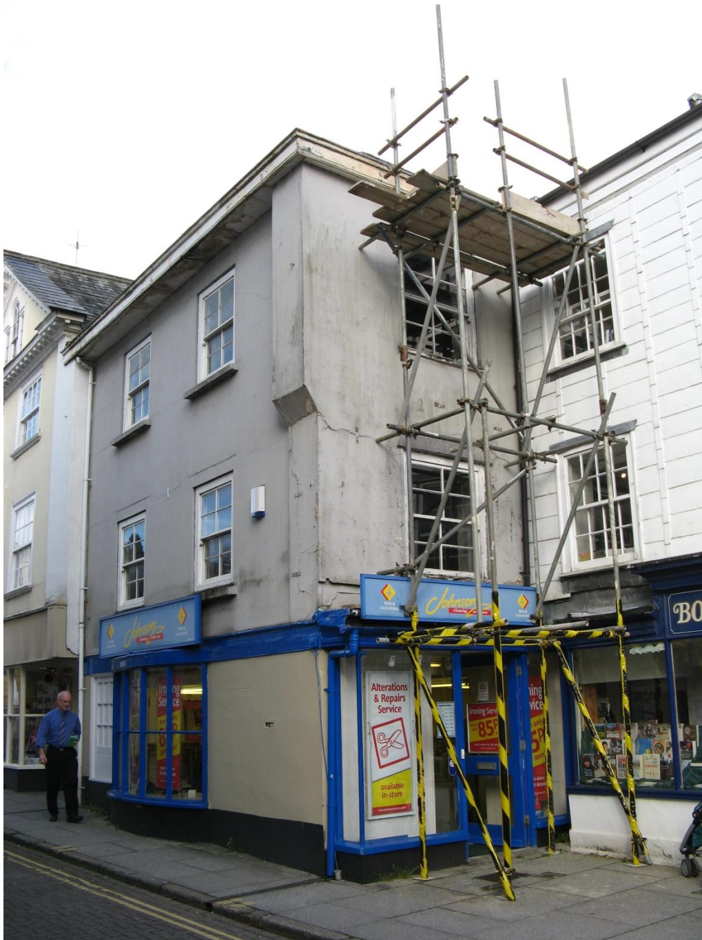
Market Street Repairs
