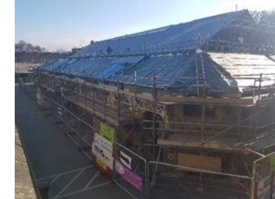
Pannier Market upgrade works
