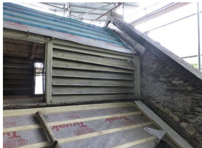
Repairs underway to the roof and windows.
