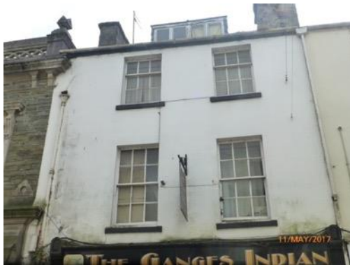
Before: The front elevation needed to be re-rendered to reduce water penetration and the internal humidity, which was a significant problem in the upper floor flats.
