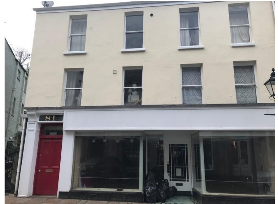
After: The reduction in height of the fascia revealing windowsills above has enhanced the appearance of the principle elevation on the street scene.
