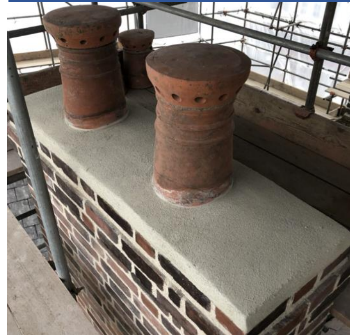
Repaired and repointed chimney on Kingdon House
