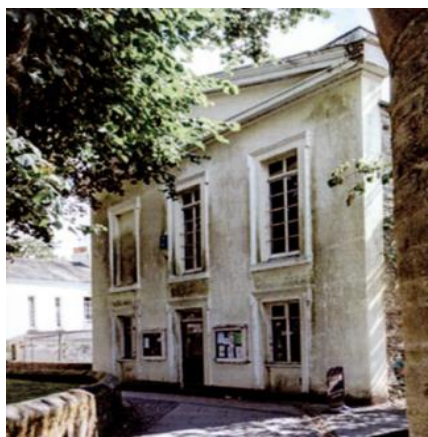
Before: Showing serious signs of dilapidation
