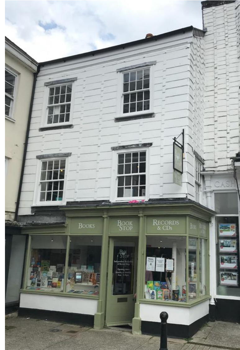
After: Completion of 3 Market Street
