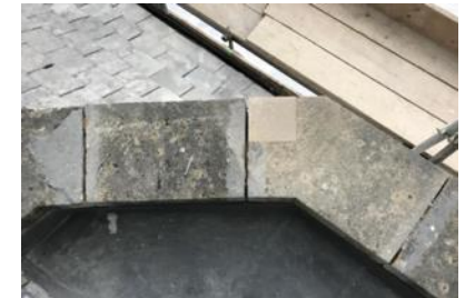
Sensitive indent repairs were made, rather than replacing the whole stone. This saved as much of the original stonework as possible.
