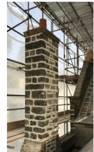
After: Repointing with lime mortar
