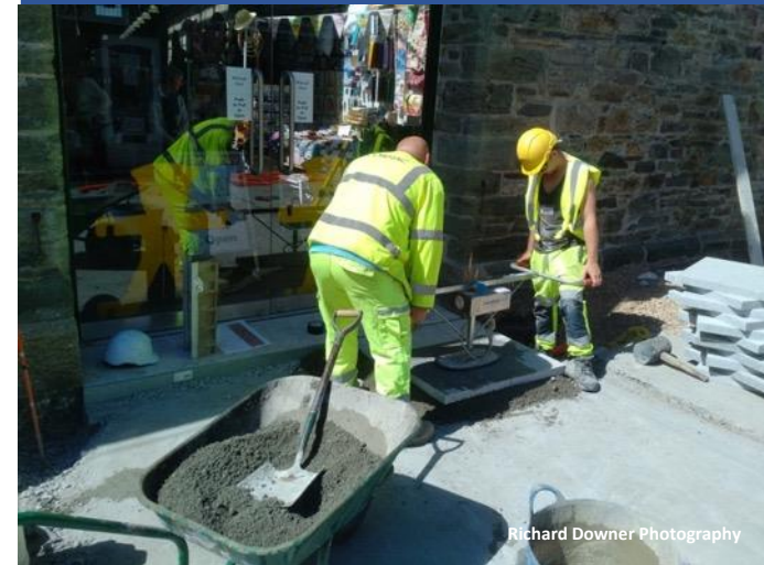
Work underway on the Pannier Market public realm project
