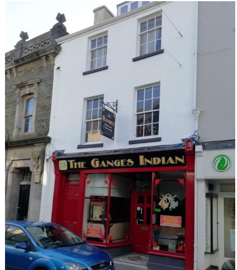
After: Isolated repairs of the timber shopfront included replacement of fluted pilasters and installation of new lead flashing on top of the front fascia, dressed into the rendered masonry wall with lead roll details.
