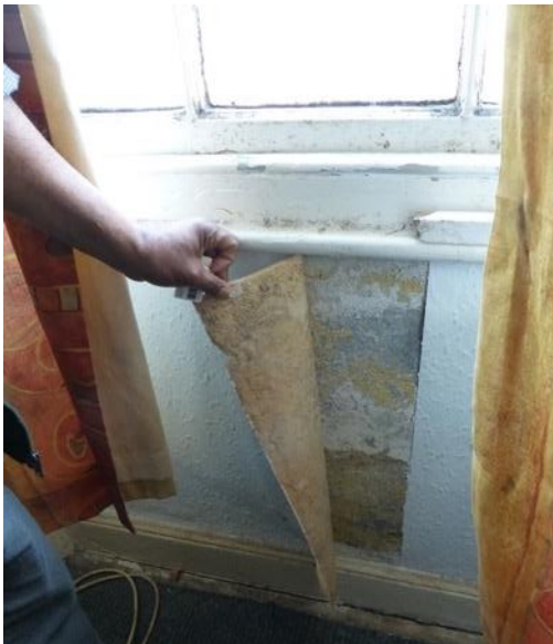
Before: The front elevation needed to be re-rendered to reduce water penetration and the internal humidity, which was a significant problem in the upper floor flats.
