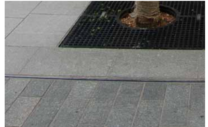
EXAMPLE OF A SLOT DRAIN
