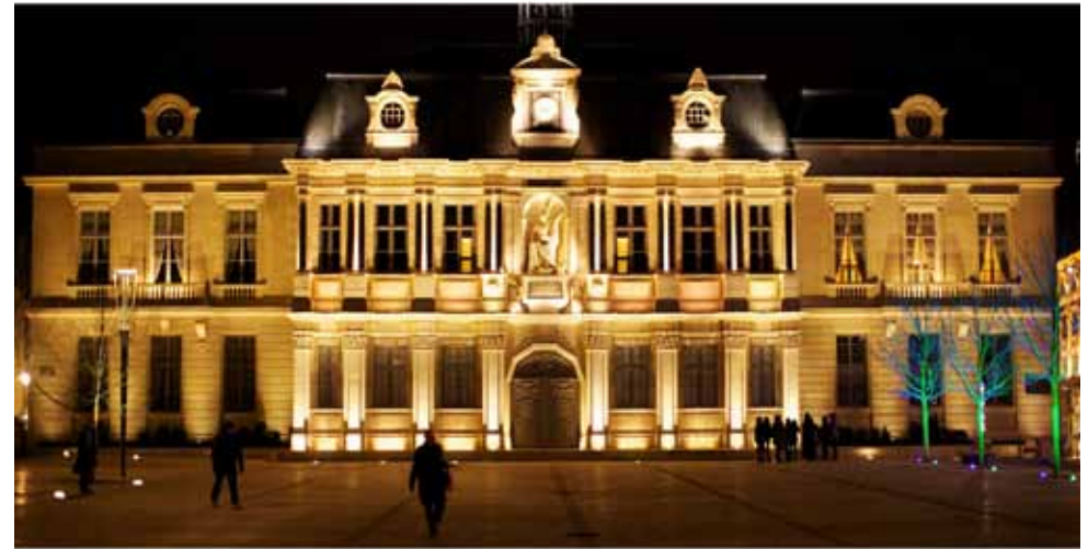
EXAMPLE OF LIGHTING WHICH MAKES THE BEST OF ARCHITURE IN THE EVENING
