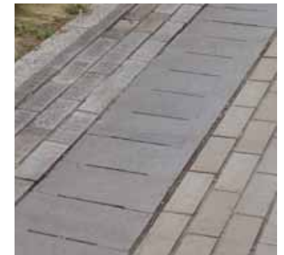
EXAMPLE OF AN INFILL CHANNEL DETAIL
