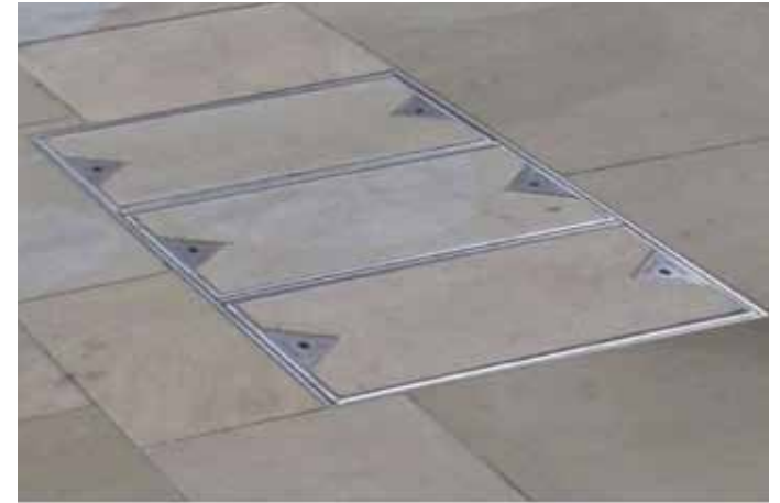
EXAMPLE OF A RECESSED INFILL SERVICE COVERS
