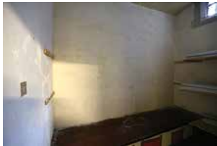
Present interior of 1892 cell
